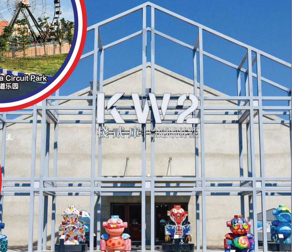
Kaoshiung Port Warehouse No.2 (KW2) KW2栈贰库
