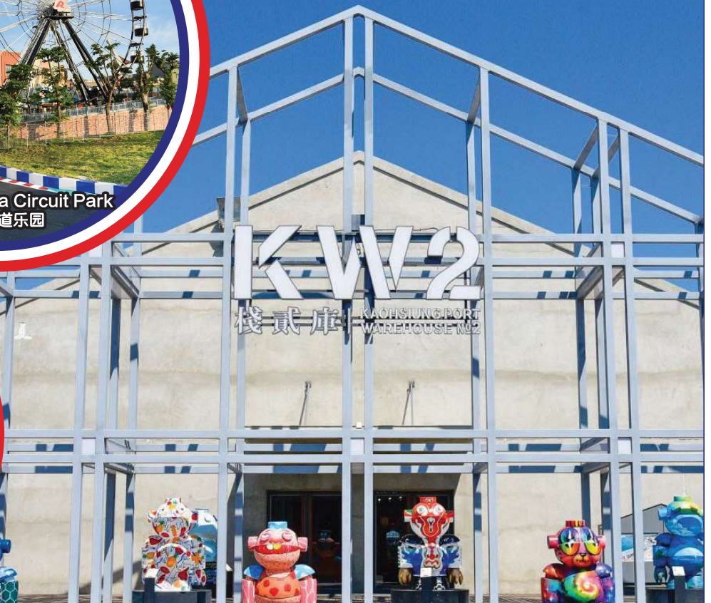
Kaoshiung Port Warehouse No.2 (KW2) KW2栈贰库
