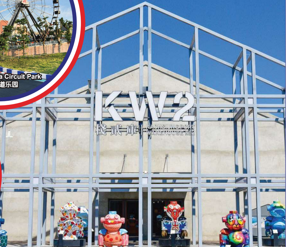
Kaoshiung Port Warehouse No.2 (KW2) KW2栈贰库
