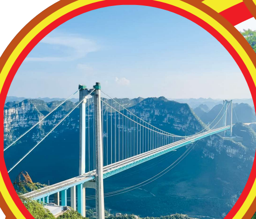
Huijiang Canyon Bridge 花江峡谷大桥
